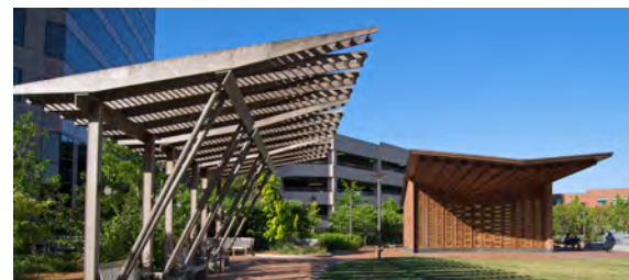
Modular Shade Structure
